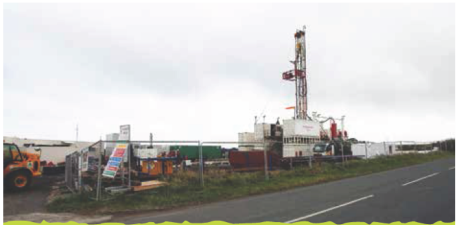
SM1 with coring rig on site
